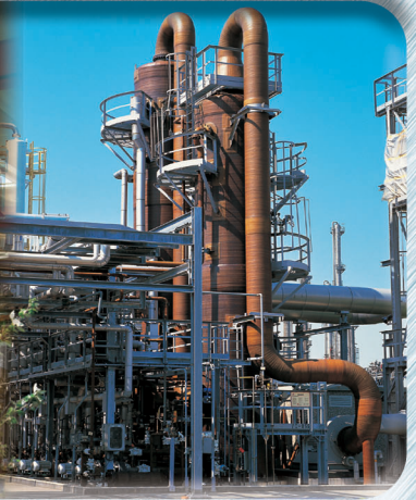
GRP Piping & Vessels
